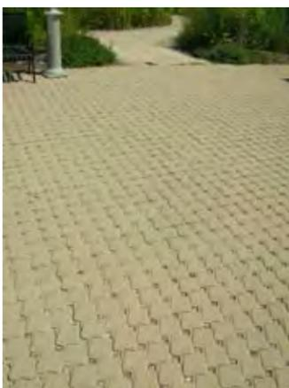
Permeable paving could be used in parking areas to offset potential stormwater issues. Coordination with the Engineering consultant will be important to understanding the benefits of this type of technology.
