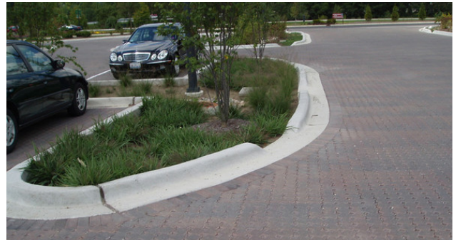
Permeable pavers combined with recessed planted islands slow surface runoff in parking lots.
