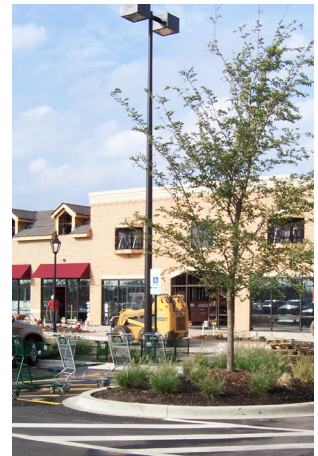
Utilitarian parking lot lighting is coordinated with traditional pole mounted lighting adjacent to the pedestrian walkway.
