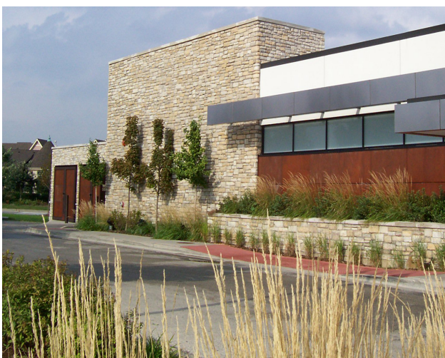
The masonry wall and wood doors of this service area are integrated into the overall appearance of the building.
