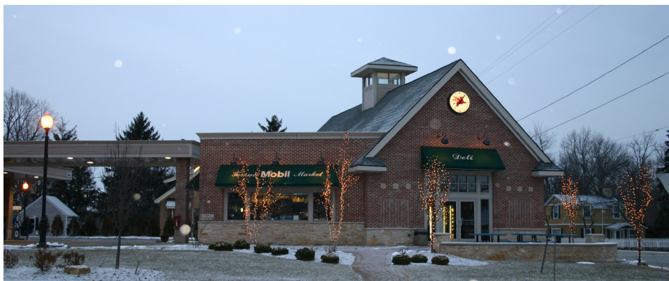
Moderate lighting is incorporated into this gas station, creating a safe and attractive nighttime appearance.
