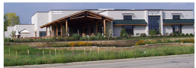
This detention basin is framed by a terraced retaining wall and landscape plantings.
