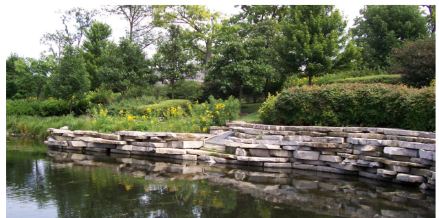
This naturalized retention pond includes stone edging and groupings of native shrubs and grasses.
