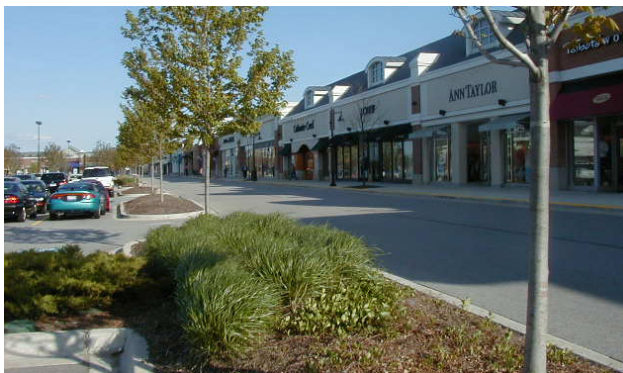
Landscaped parking island reduces the amount of pavement and provides automobile screening.
