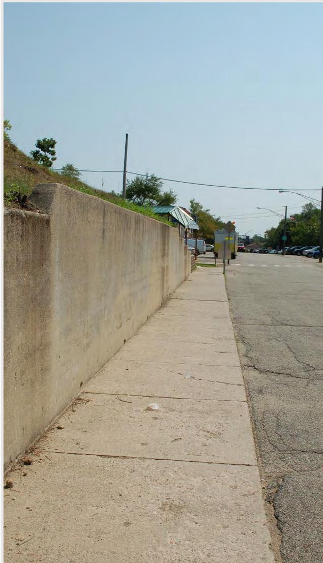
This image shows a detail of the concrete retaining wall and deteriorated sidewalk. These elements combined with the lack of separation from the street and the lack of street trees and lighting, contribute to a negative pedestrian experience along the east side of Nippersink Boulevard.
