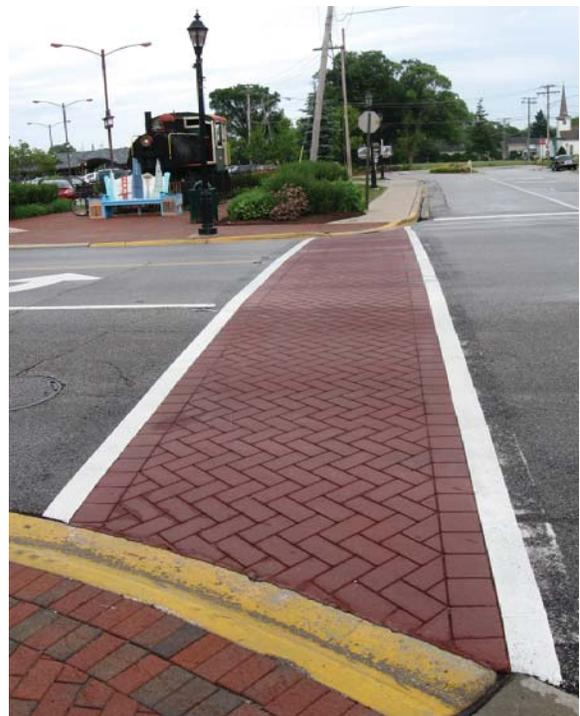
Suggested Pedestrian Crossing using color thermo-plastic inlay into asphalt pavement
