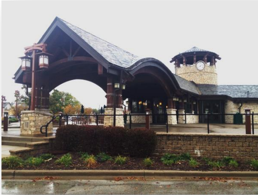
Tinley Park Metra Station. Photo Credit: RTA
