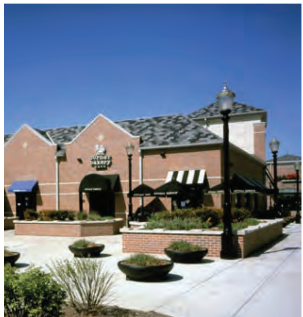
Outdoor dining plaza is defined by paving and site furnishings
