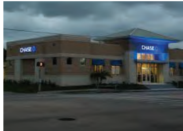
Building lighting is designed to highlight major building features and minimize light trespass.
