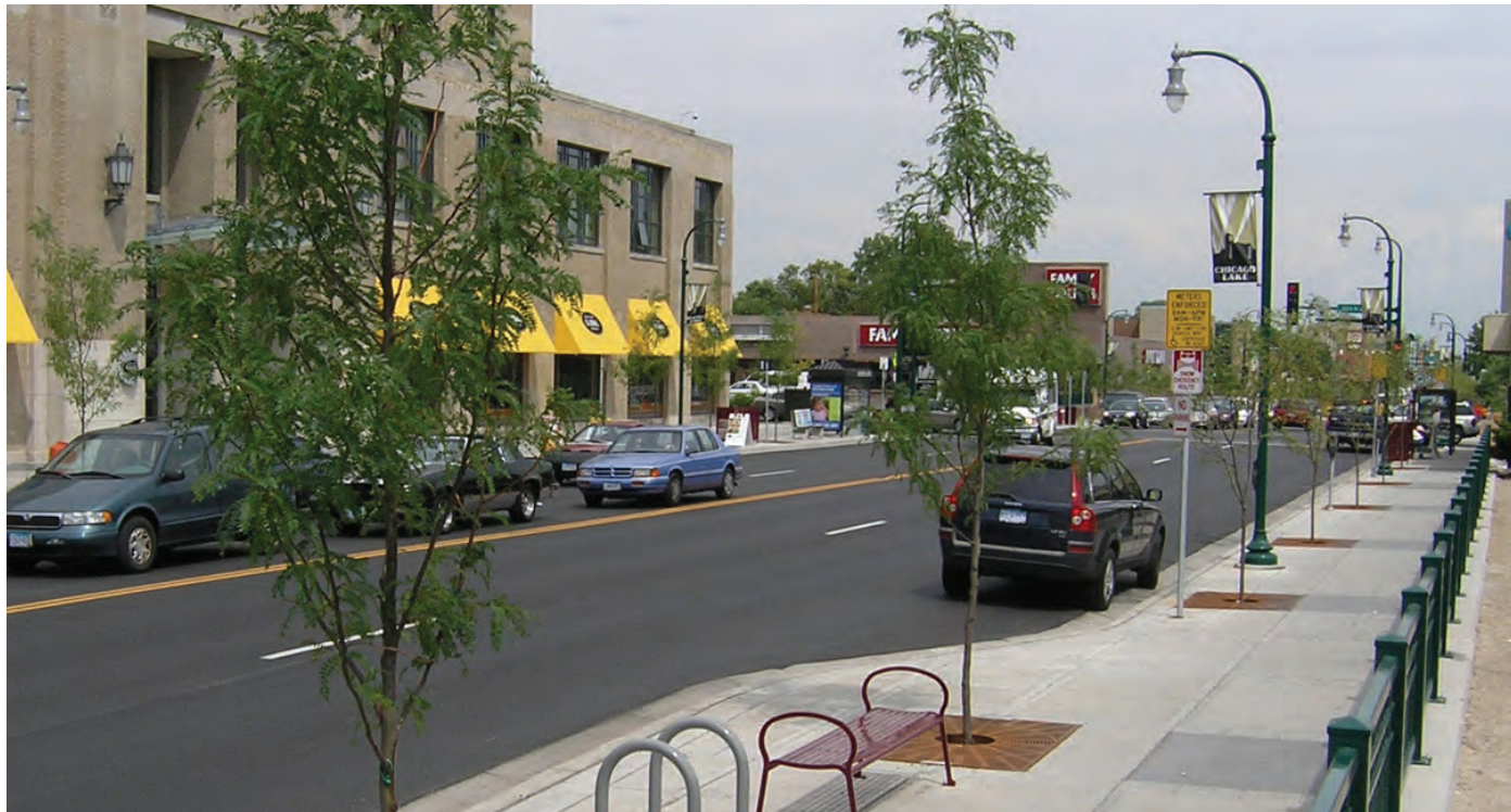
Curb bump-outs, widened sidewalks, street furnishings, lights and tree plantings support a pedestrian friendly streetscape that would enhance on-street parking in Chicago Ridge and interior roadways of development sites
