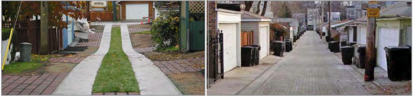
To ensure residential alleys do not create a “sea of asphalt”, sustainability techniques such as the introduction of grass patches (left) and pervious pavers (left and right) can be used to help integrate more natural elements into the alleyway and provide better stormwater management for rainwater runoff.
