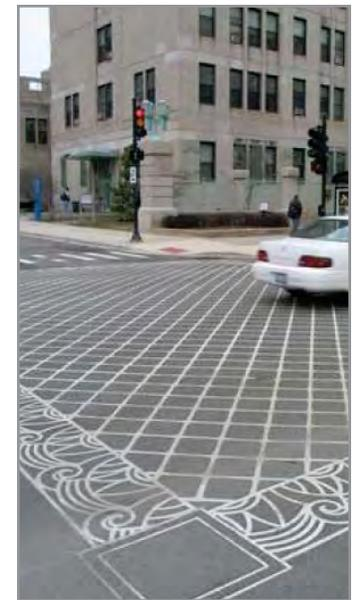
While colored or brick pavers are often used to accentuate the streetprint of an intersection, the use of Duratherm paving can also be used as an alternative to create a unique character to the street. Duratherm is uniquely formulated thermoplastic material that can be inlaid into imprinted asphalt. Since it is slightly recessed below the asphalt surface, Duratherm is highly durable and resistant to wear caused by auto traffic. Different colors and patterns can be utilized in a Duratherm design.
