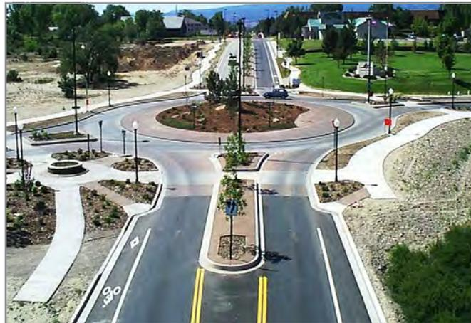
*While facilitating auto traffic flow, a modern roundabout can integrate elements such as bicycle lanes, paved crosswalks, pedestrian-scale lighting and planters, medians, and landscaping.*
