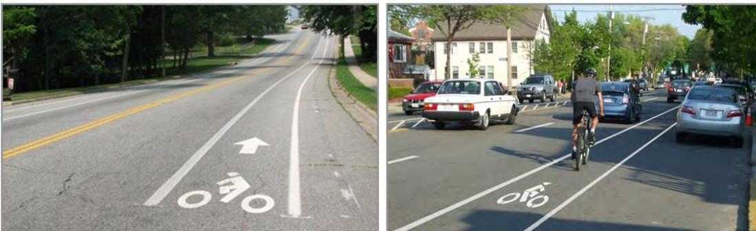
Rather than being separated from the roadway like off-street paths, marked bicycle lanes are delineated on the roadway with clearly painted markings and directional indicators. In the left image, the bicycle lane is located between the vehicular travel lane and shoulder. The right image is similar except the shoulder is replaced by parallel parking. In both cases, a sidewalk is provided in addition to the marked bicycle lane.
