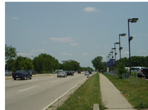
Eastbound Lincoln Highway/US Highway 30
