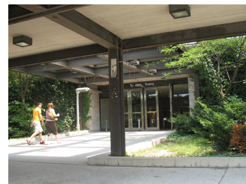
Station house exterior
