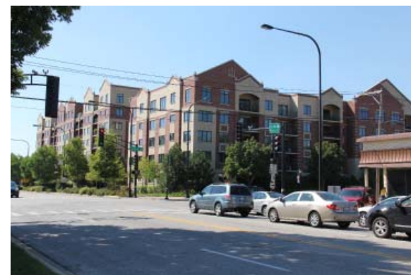
Looking southwest on Route 83 at Central Road
