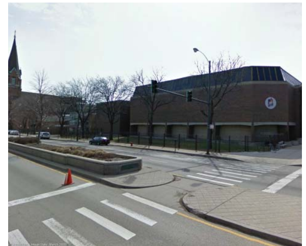
Landscaped median with pedestrian refuge
