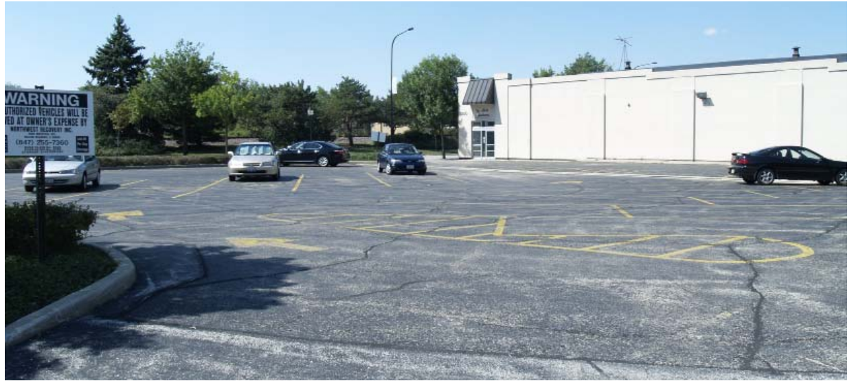
Existing Tri-State Site
