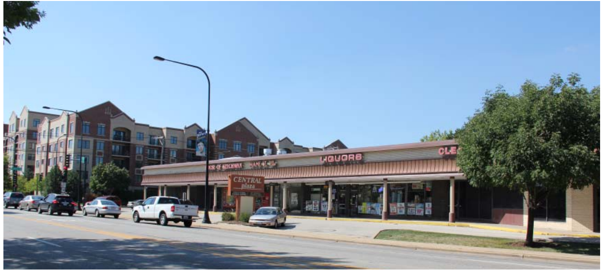
Existing Central & Main Site
