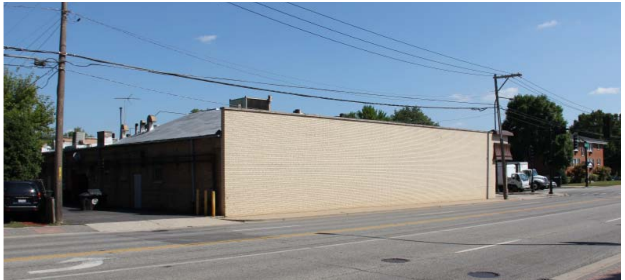
Existing Central & Main Site
