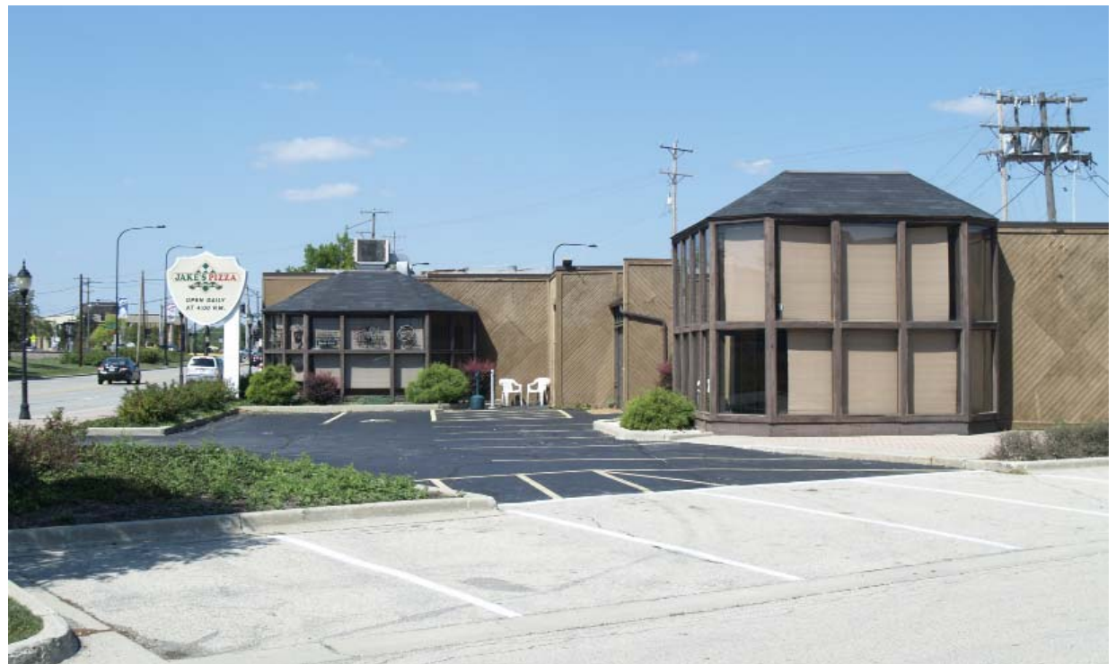
Existing condition of Jake's Pizza parking lot - viewed from Elmhurst Avenue
