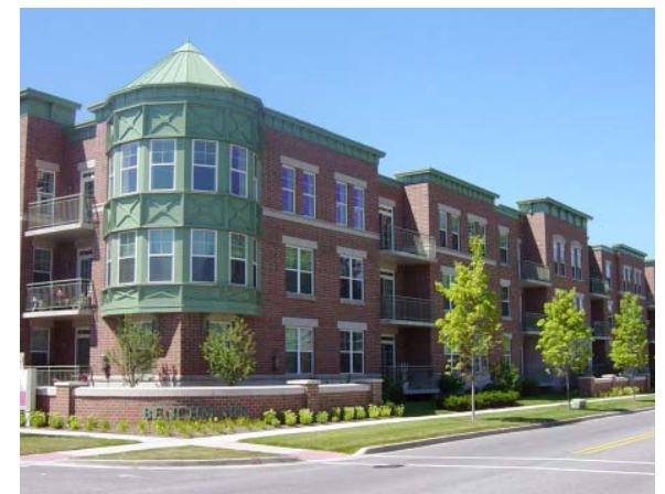
Smaller buildings provide a transition into surrounding areas
