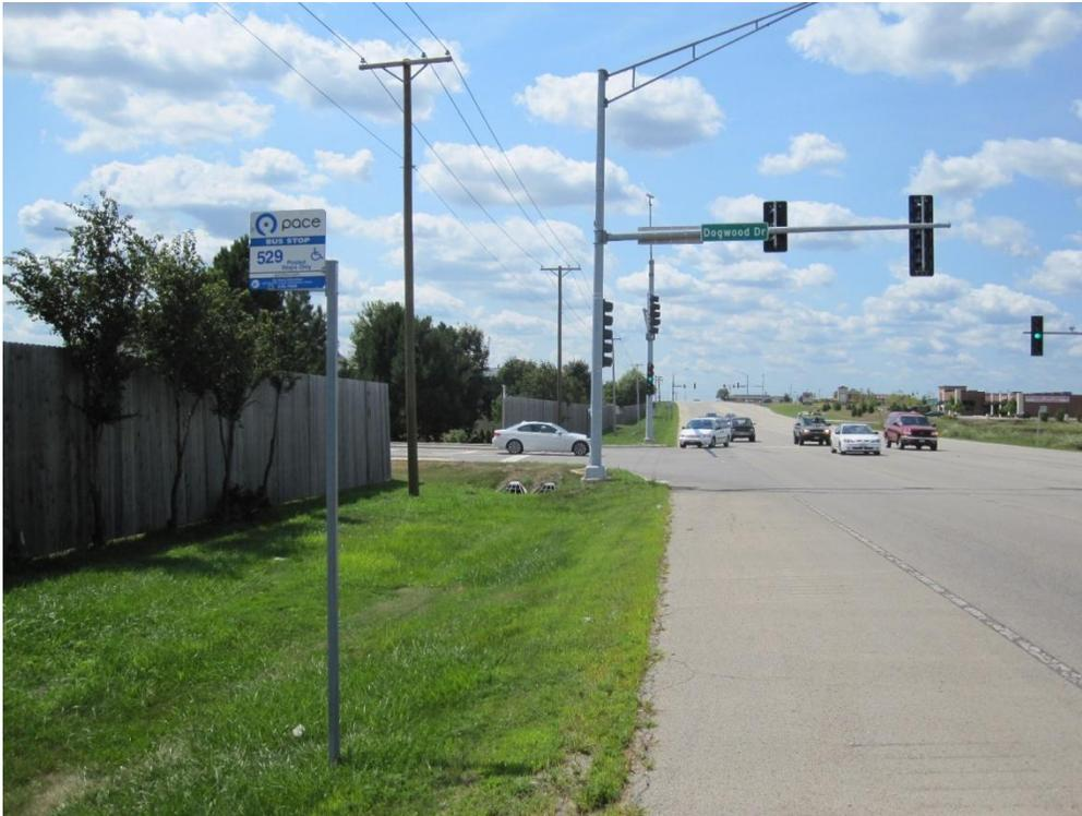
This treatment does not represent a suitable ADA accessible route as it is not separated from the roadway nor does it provide a dedicated walkway. In many cases, roadside shoulders are typically designed to slope away from the roadway at a 4% cross slope to better drain surface runoff. This is an unsuitable cross slope for the disabled to traverse. For the stops at Sullivan Road, the shoulder is loose gravel and thus entirely inaccessible to the disabled.
