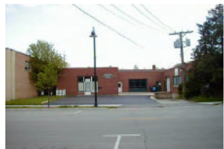
Building to site relation is poor. Prevailing setbacks are not maintained.
