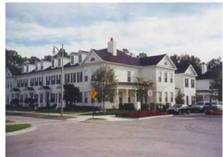
Balconies, setbacks, and projections can be used to give the appearance of a collection of smaller structures.
