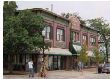
Example of building incorporating shutters, lintels and a strong cornice line. The use of vertical elements to minimize mass should also be noted.
