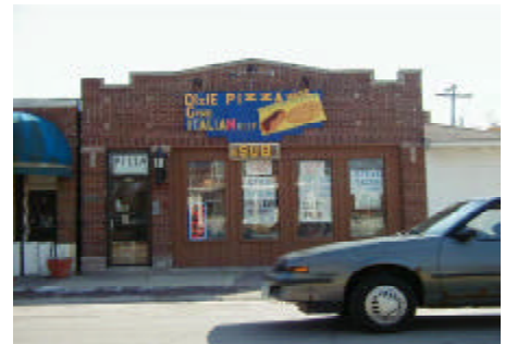
Signs have poor relation to building architecture and color.
