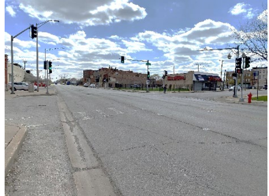
154 th Street at Park Avenue Intersection (looking south): pedestrian signals are present, but crosswalks are limited and pedestrian crossings are incomplete.
