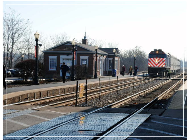
MD-W Train entering existing Elgin Metra Station
