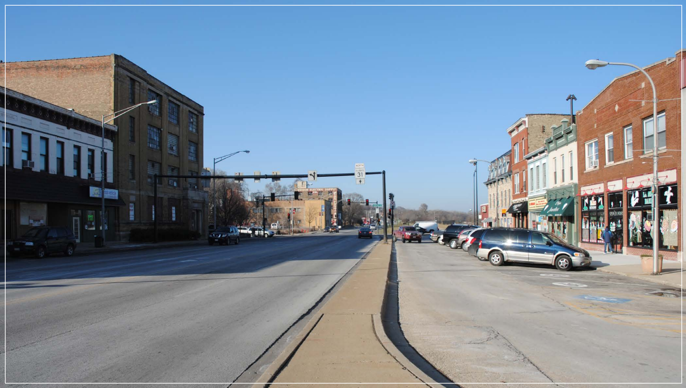
View north on State Street just south of Chicago Street - Current Conditions
