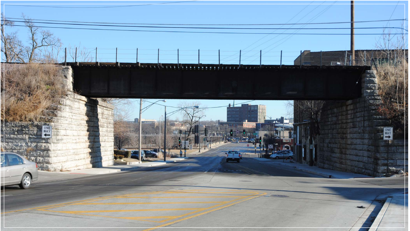
Highland Avenue Underpass - Current Conditions
