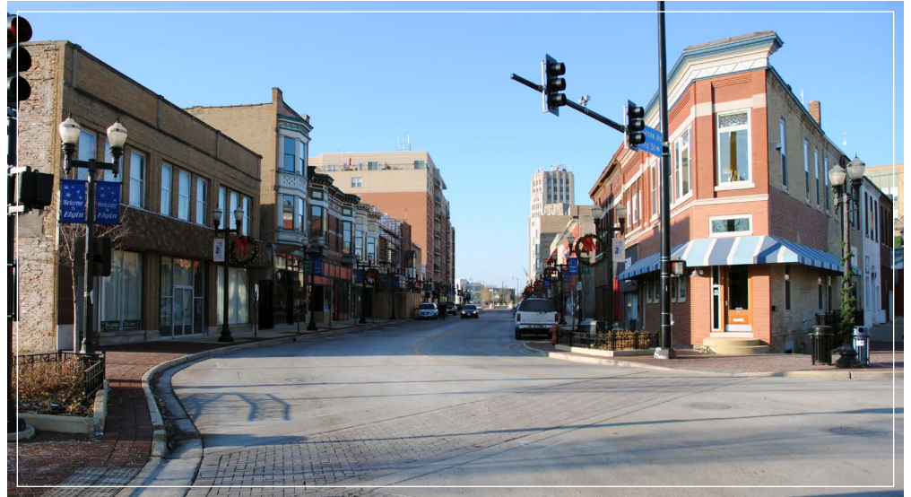
Building maintenance and facade enhancements south of Fountain Square
