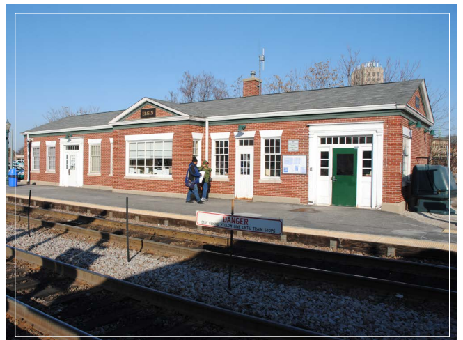
Elgin Metra Station - Existing Facilities
