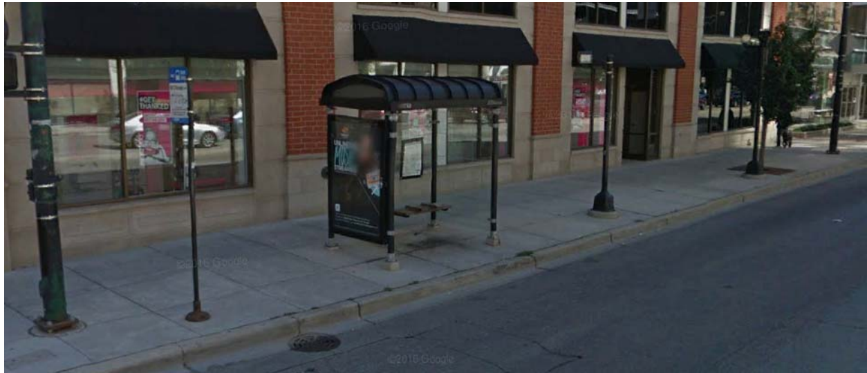
Figure 6: Northeast Corner of Chicago - Clark Bus Stop and Shelter
