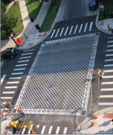
Define crosswalks by incorporating alternative paving materials (above), and provide bumpouts (below) at corners where they will not interfere with bus movement.
