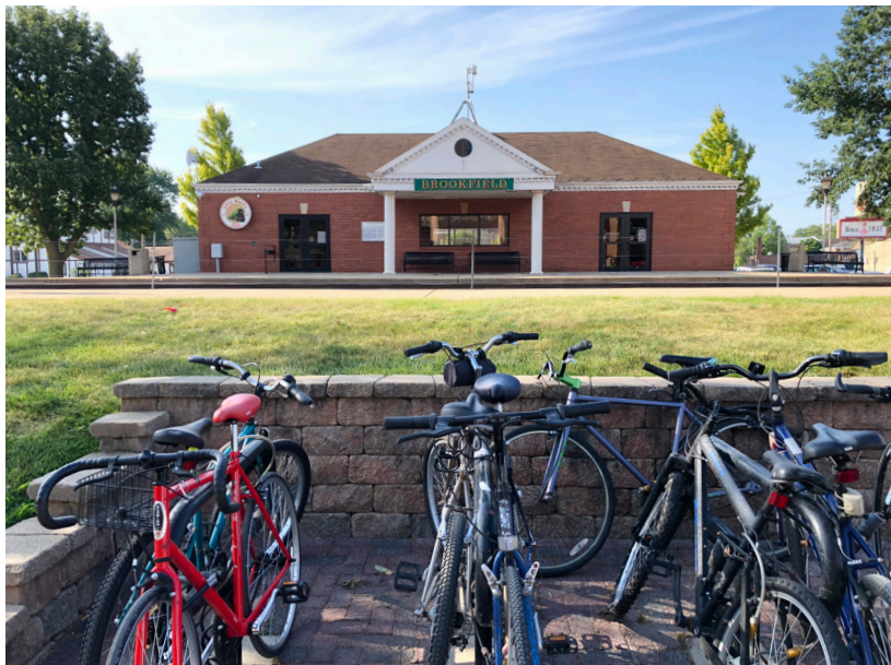
Brookfield Metra Station
